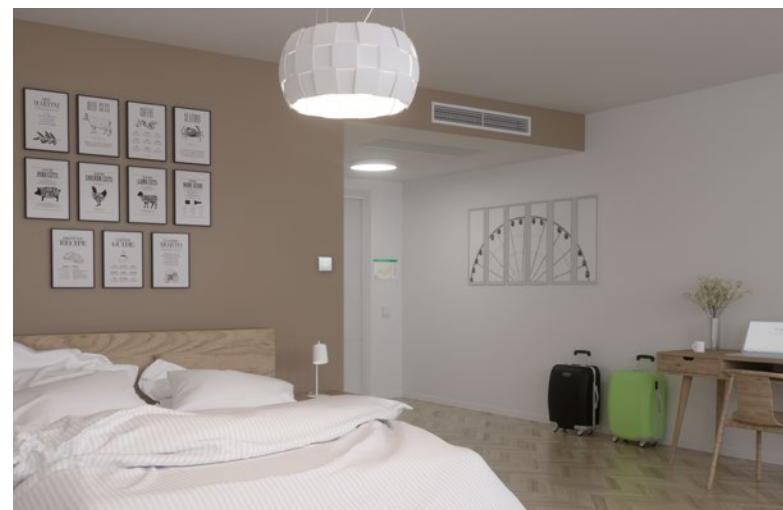
Hotel room with setpoint selector switch, waterborne cooling and heating as well as demand-controlled air regulation. Key card holder for occupancy.
