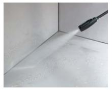
Cleaning with a chemical solution is possible due to PET inner wall lining and sealant with a hygiene certificate
