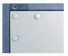
Unit wall is weather and UV-resistant, consisting of a composite frame construction and composite panels with a gel-coat top layer.
