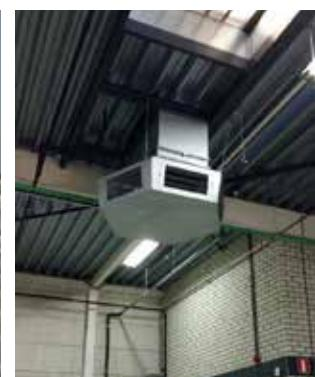
Winter cover      6-sided hexagonal air blowing plenum with horizontal louvres
